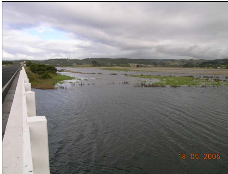
Picture 1. Barham River backwater inundation in the vicinity of the proposed development.
